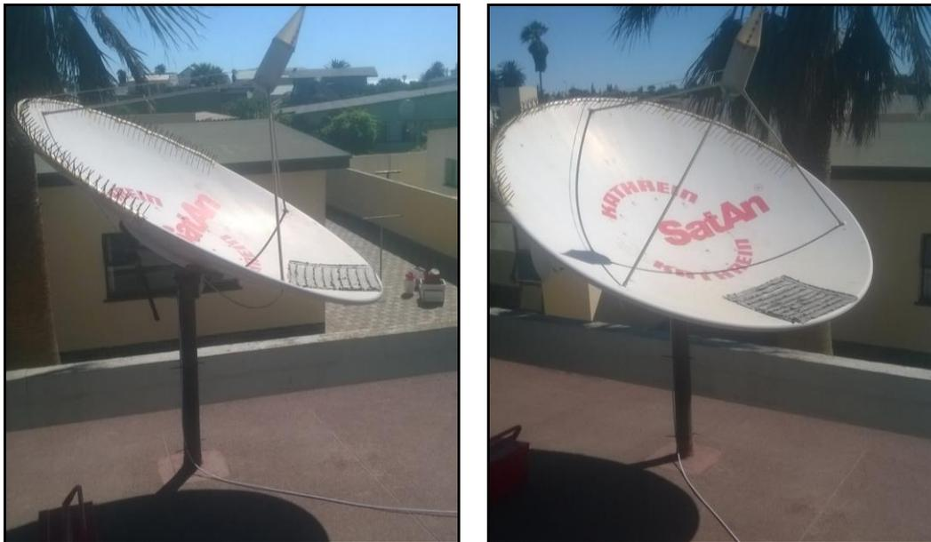
Figure 4 - Centre Focal Dish examples of an actual Satelio installation
